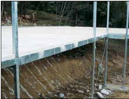
Fig 1.1 Residential Suspended Ground Floors
