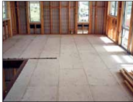
Fig 1.2 Residential Suspended First Floors
